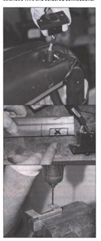
6 If you started with electric SN-95 seats, remove two screws, a few tiedowns and then the controller itself (top). You will reuse this harness. To mount the switch to the new Flofit seats, you'll need a bracket. Mark a piece of angle aluminum (available at any hardware store) like so (middle), and then cut the hole with a hacksaw or chopsaw. Be sure to clean up the edges so as not to get cut. Drill two holes for the switch screws and two more to attach the bracket to the seat.
